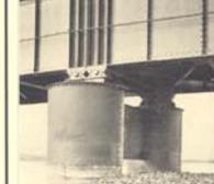
**EXPANSION BEARINGS** are best maintained with NO-OX-ID. The vehicle in NO-OX-ID being a petroleum product, the dual service of rust prevention and lubrication are obtained through its use.
