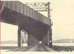
**THE STRUCTURE** pictured above is subjected to accelerated corrosion from locomotive gases.
